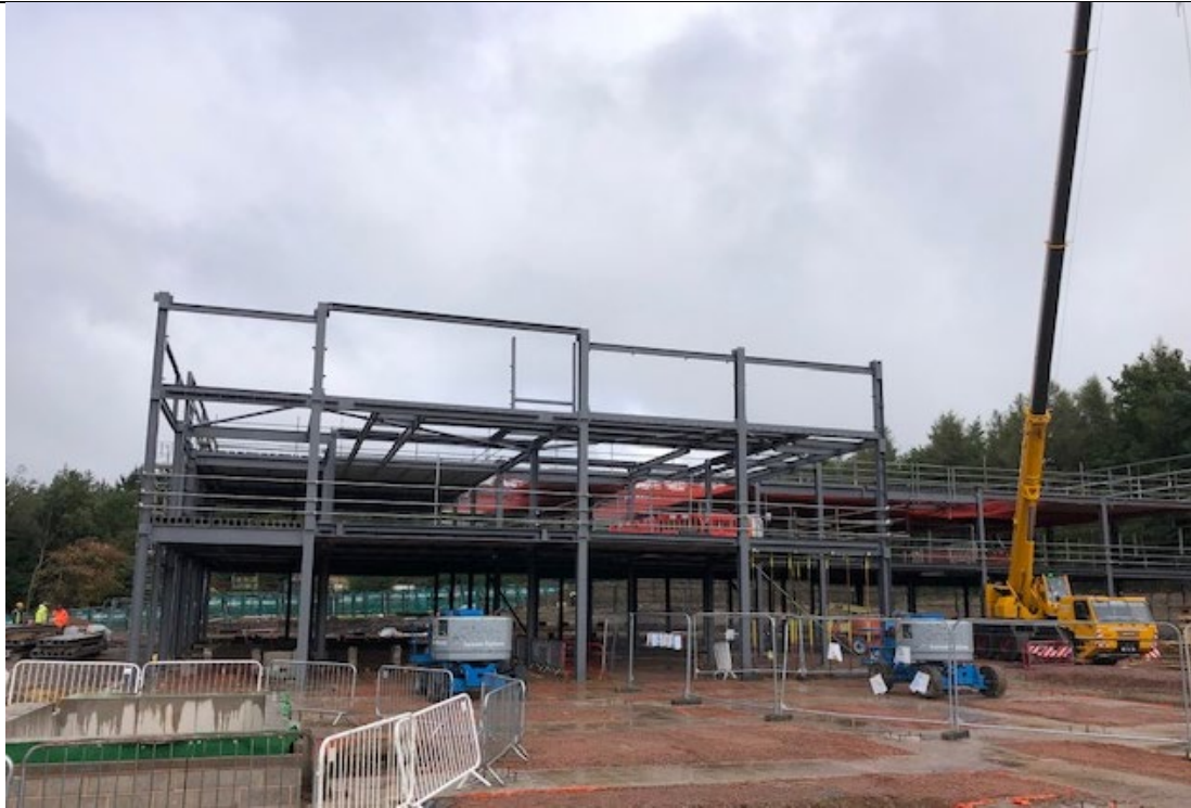
Phase 1 & Phase 2a steel frame & concrete plank installation
