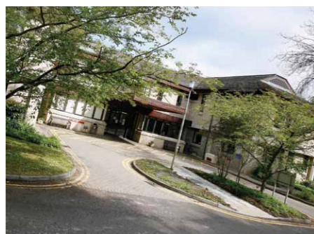
Completed refurbishment at Cirencester Minor Injuries Unit
